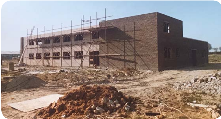
Pickering Electronics building being built in 1979.
